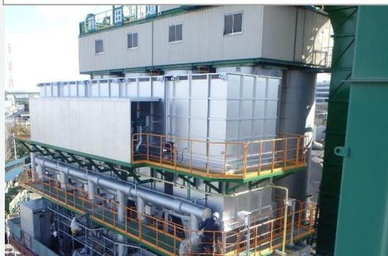
Thermal storage and combustion type odor furnace at Asaka mixture plant
