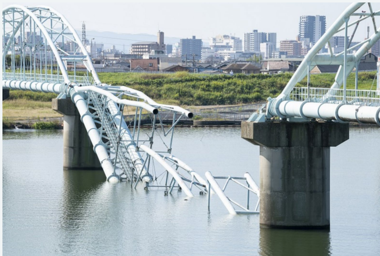
Collapse of the Rokudo Water Pipe Bridge in Wakayama City resulted in water outages for about 60,000 households
